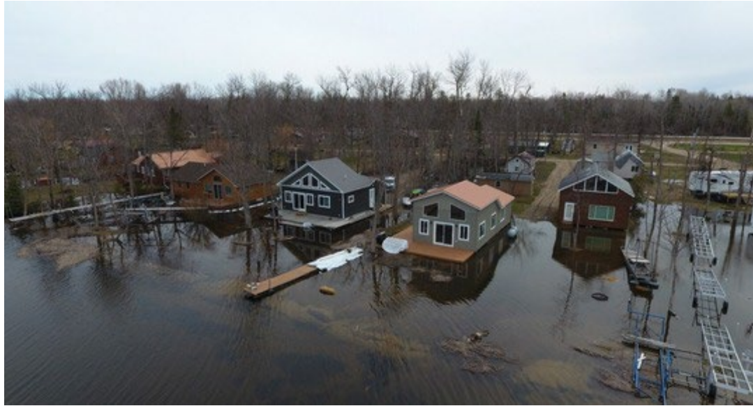
Lakeshore flooding, spring 2019. Photo credit: HDR.
