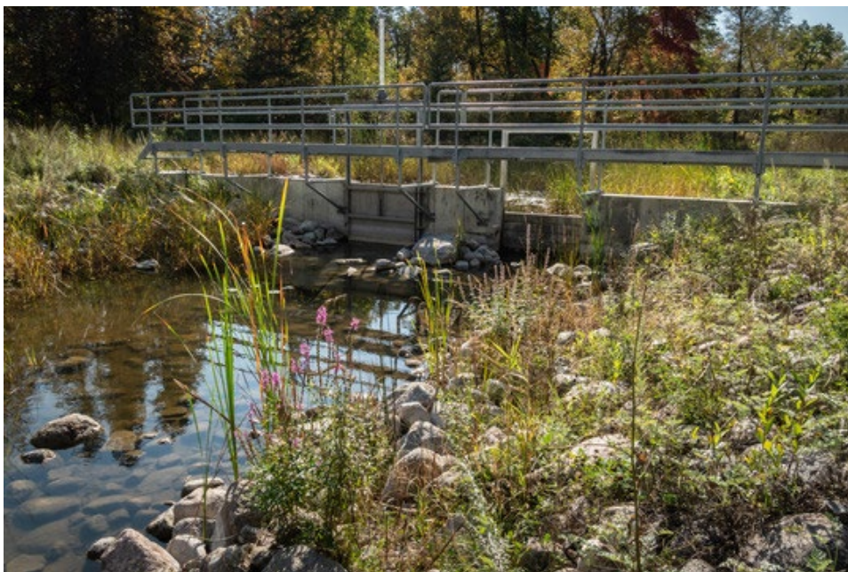
Pine Lake outlet gate from downstream side. The rock arch rapids are outside the photo to left. Photo credit: Janet Nelson.
