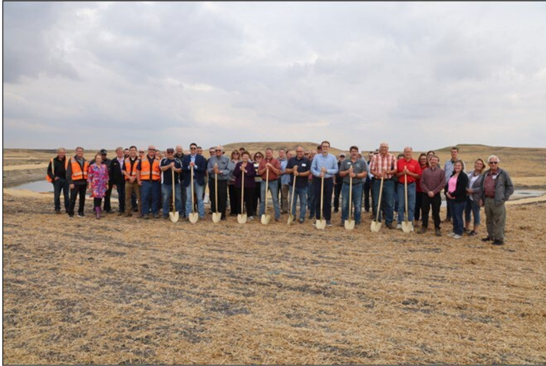
Participants at the groundbreaking ceremony on the Mustinka River. Photo credit: Moore Engineering.
